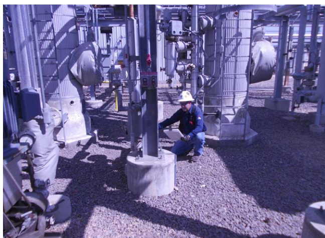
Figure 2. Mechanical integrity field data collection being gathered for TIR’s data management team to analyse and process.
