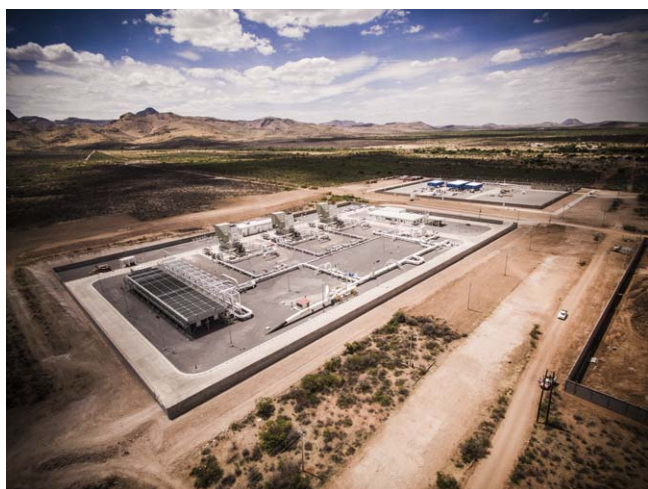
Figure 2. El Encino is the largest natural gas compression station in Mexico territory with a total of 155 000 hp of mechanical power installed on site.
