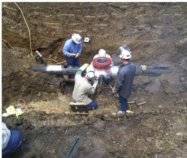
Figure 1. Pipeline split tee repair option. TIR supports with AWS certified Weld Inspector, NACE coating inspection and utility inspectors. API 1169 certified options available.
