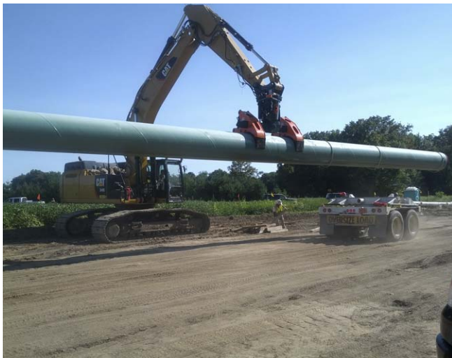
Figure 2. Safely, precisely and efficiently stringing the ROW.
