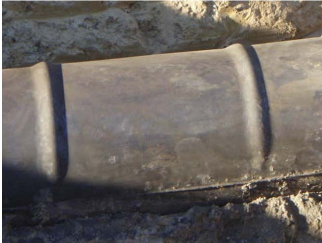
Figure 1. Exposed wrinkle bend 1 .
