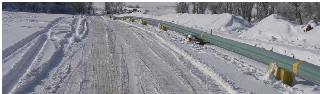
Figure 5. Regional bottlenecks and construction demands have pushed seasonal limits.
