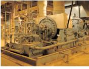
Feedwater Booster Pump for Nuclear Power Plant Model 600 X 400HDRM
