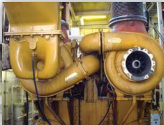
Before: ABB VTC-254 turbos installed on CAT 3612 diesel engine
